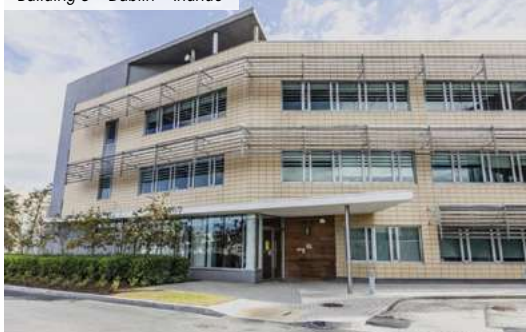
Building 8 – Dublin – Irlande
