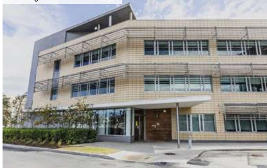
Building 8 – Dublin – Irlande
