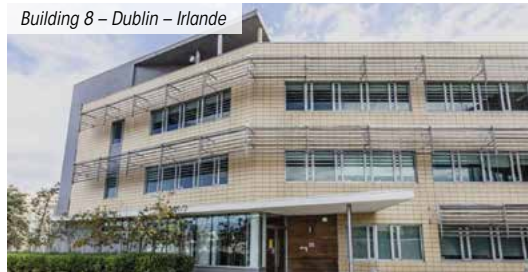
Building 8 – Dublin – Irlande
