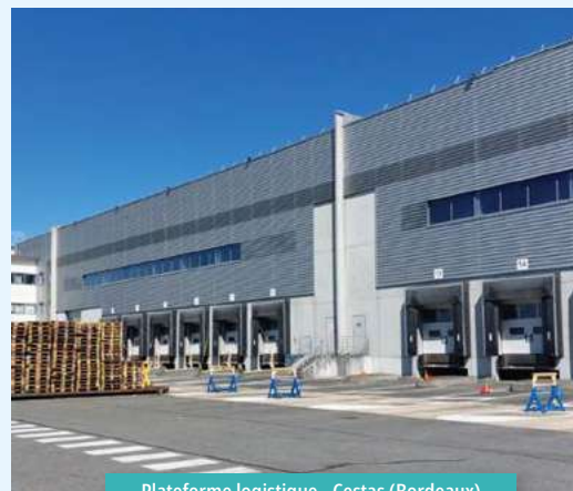
Plateforme logistique - Cestas (Bordeaux)
